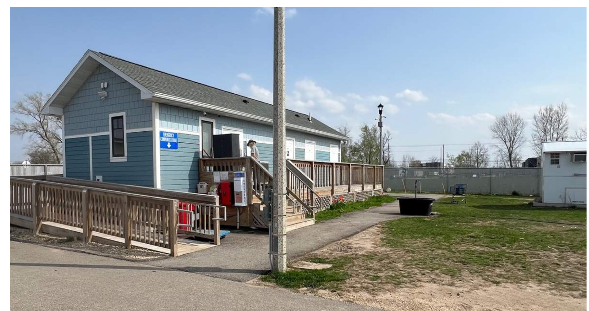
EXISTING BATHROOM/OFFICE BUILDING
