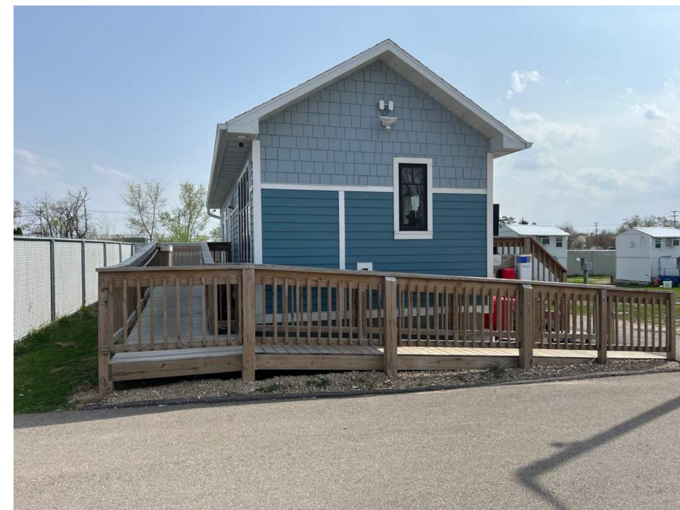
EXISTING BATHROOM/OFFICE BUILDING
